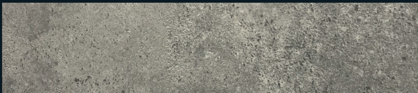
VT SOM23070 / Concrete Width: 4 m
